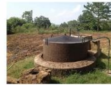
Gobar Gas Plants Cattle dung is fed to Plant Gobar Gas and Slurry Produced
